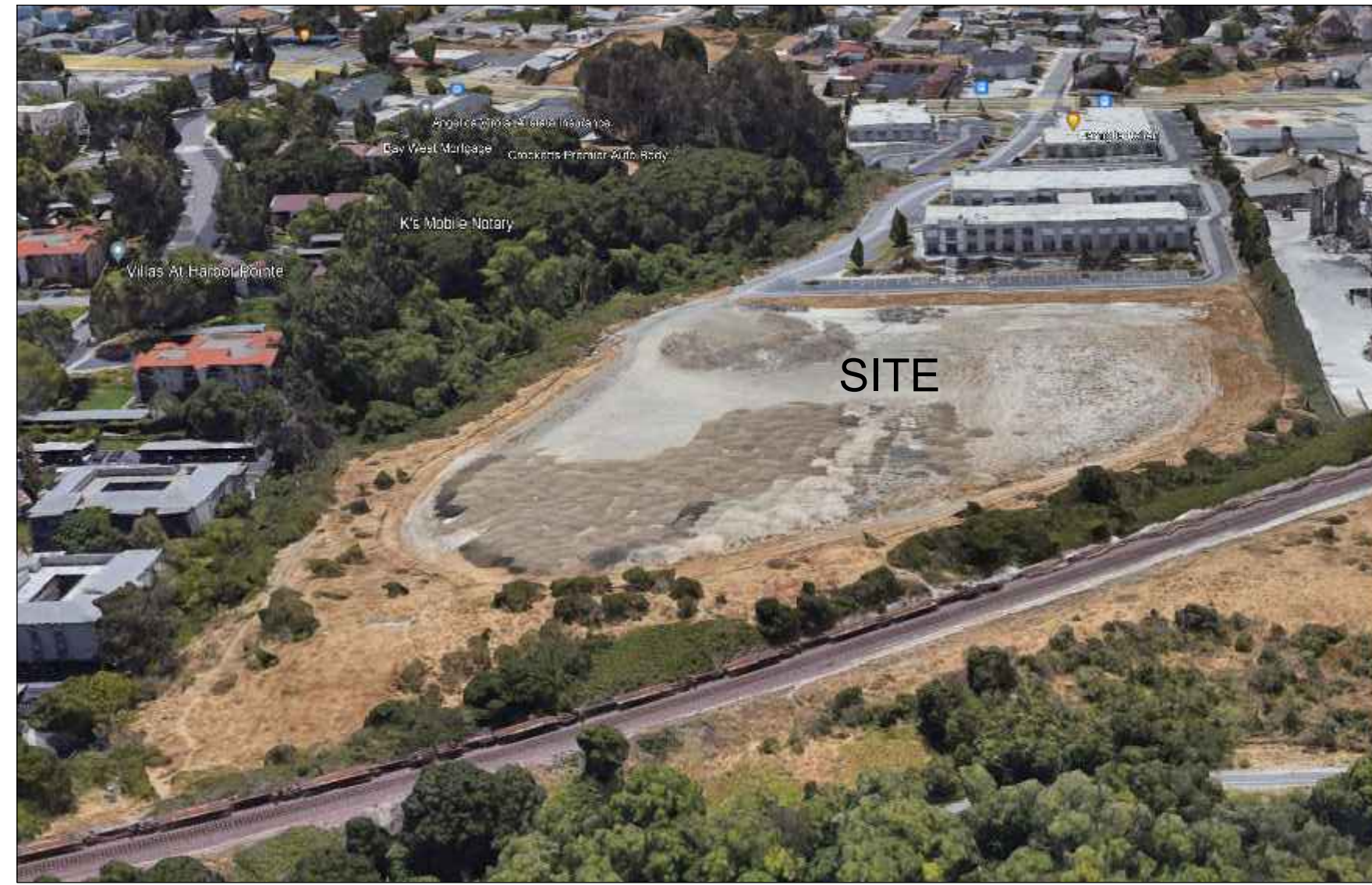
NORTH AERIAL VIEW - 2
